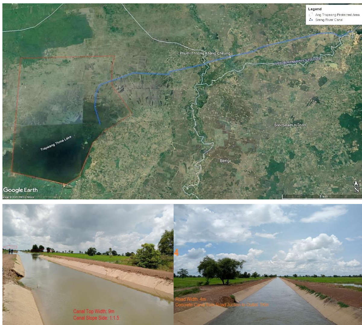
Figure 6: Sreng River canal diversion
