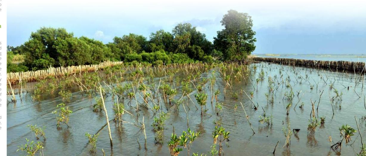
created a natural protection for the dyke toe and for recruiting mangroves. The inundation periods of near-dyke areas have been considerably reduced, and so is the maximum wave height at the dyke toe.
