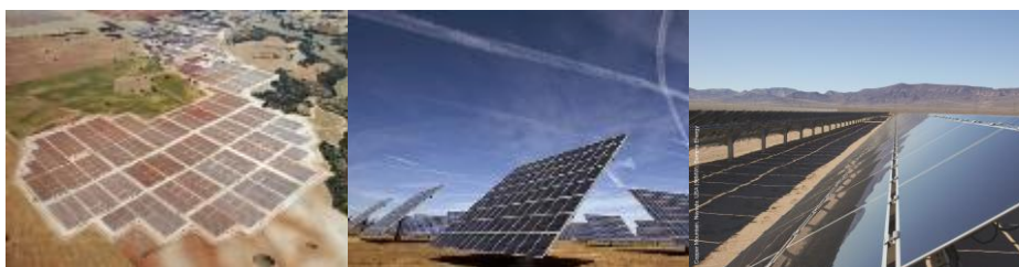
Figure 6: Fixed-tilt and tracked c-Si PV plants, Thin Film PV modules and tracked CPV plant
