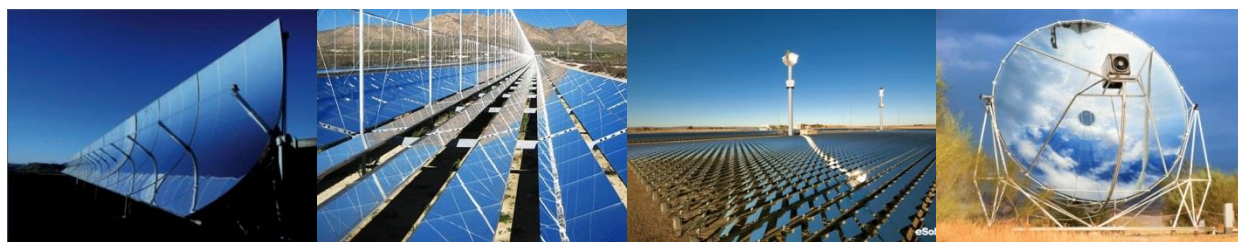
Figure 2: Line focusing systems: Parabolic Trough collector and Linear Fresnel Collector, Point focusing systems: Solar Tower plant and Dish Stirling collector.
