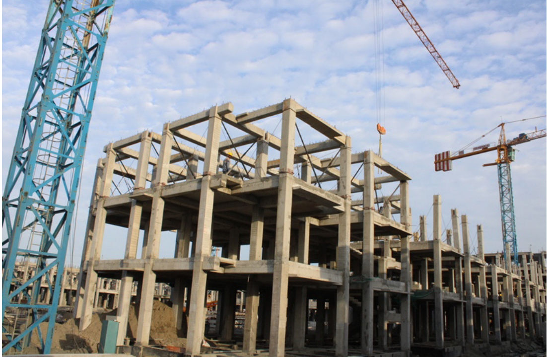
LHP project site in Chennai
