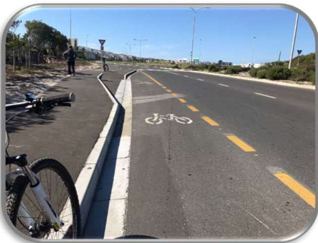
Figure 5-9: Bicycle lane developed in existing road shoulder
