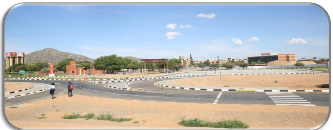
Figure 4-2: Complex pedestrian crossing environment at roundabouts along Independence Avenue
