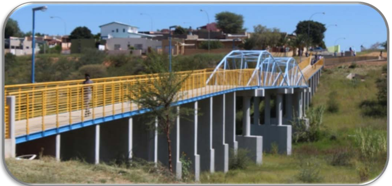
Figure 5-10: Pedestrian bridge across Arrebusch River, Windhoek
