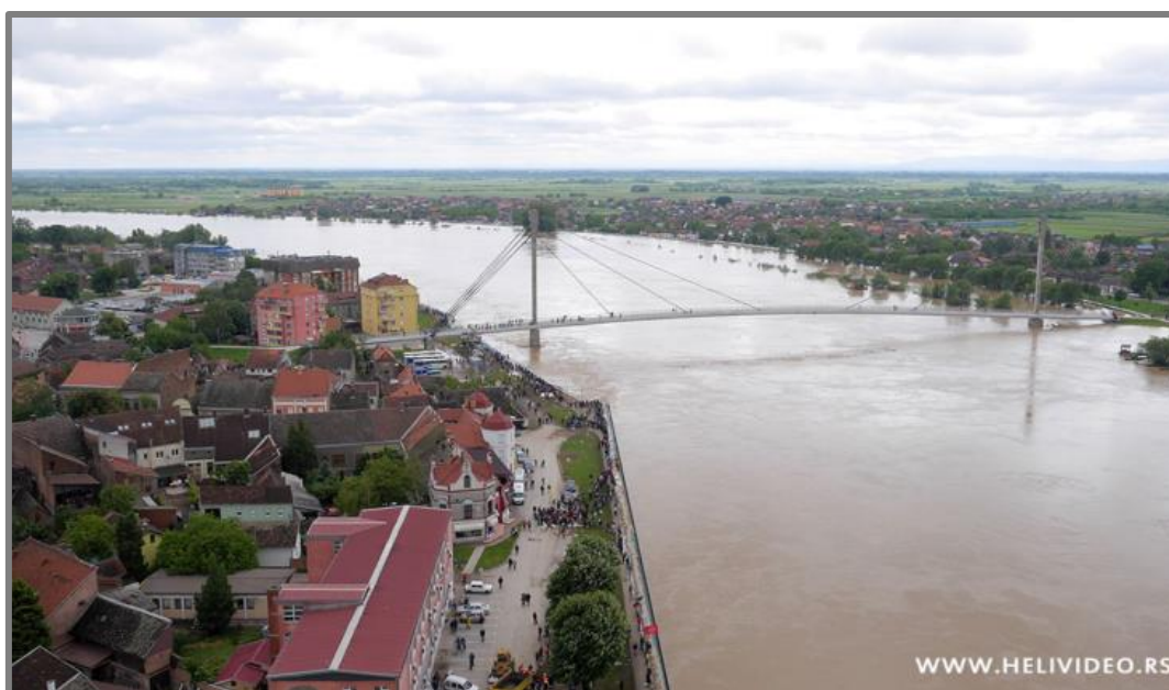
Sremska Mitrovica just before the breakdown of the embankment upstream in Croatia (Source: www.helivideo.rs )
