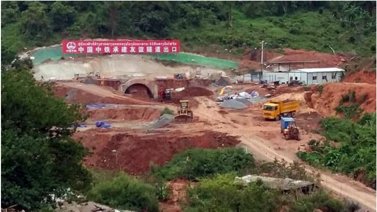
Figure 12. Photo of construction work
