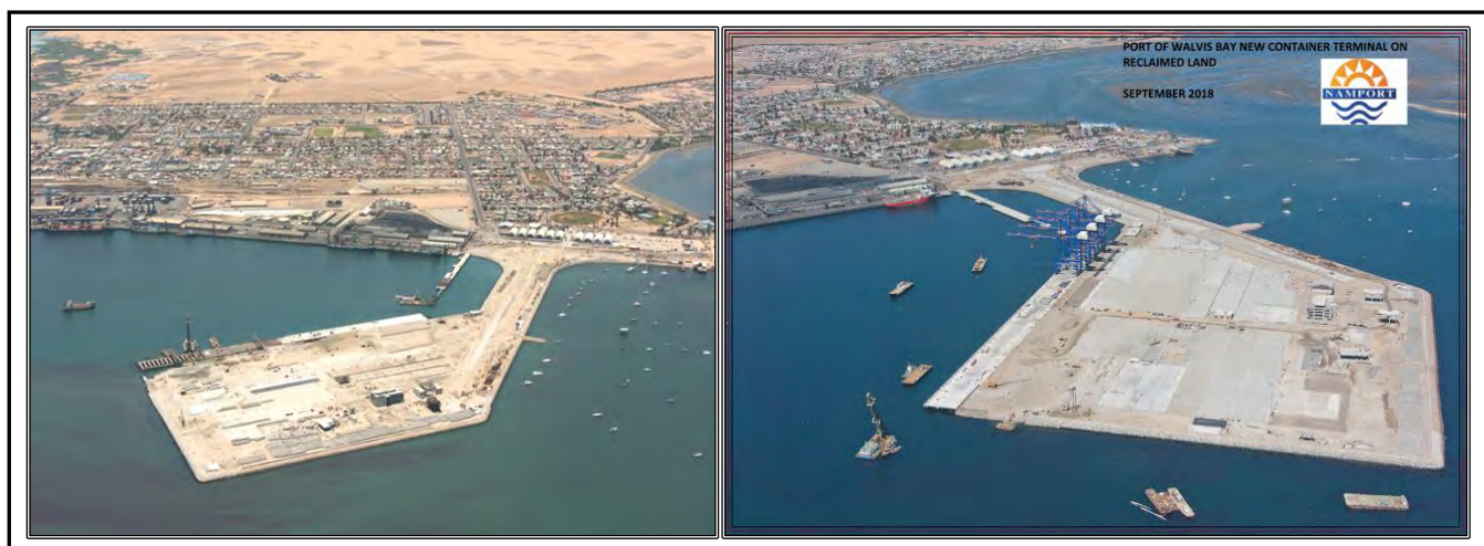
Figure 18: Walvis-bay port showing the container terminal built on reclaimed land. Source: P. Mupupa, Namport, July 2019
