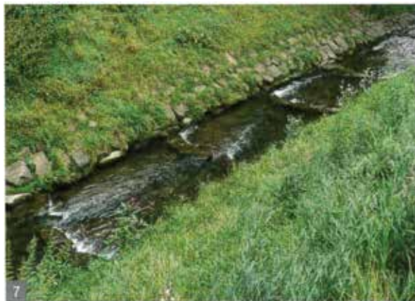
Figure 23: Steps in the river bed to increase the oxygen in the water
