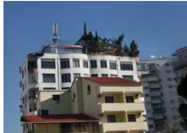
Figure 28: Example for greening of roof tops (Tirana City)
