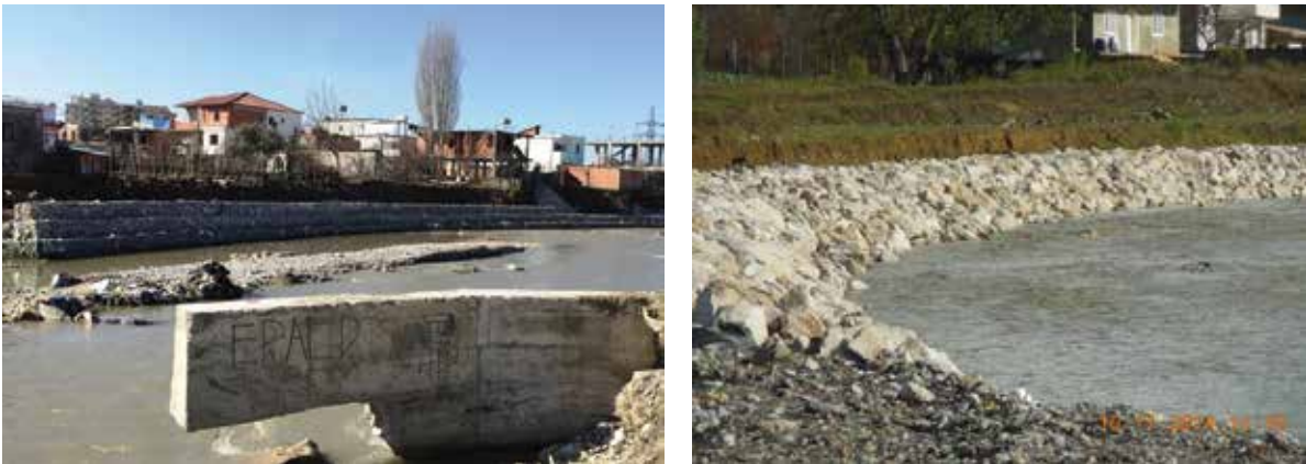
Figure 36: Flood protection measures (protection of riverbank from erosion)
