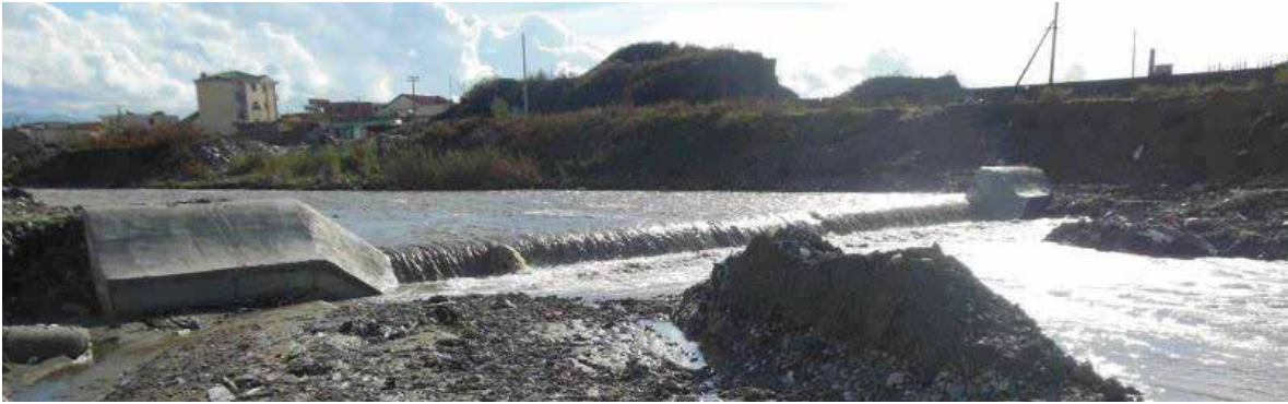
Figure 35: Construction of weirs for water retaining pool structure
