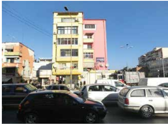
Figure 26: Situation at the cross-road in case study area 3 (I)
