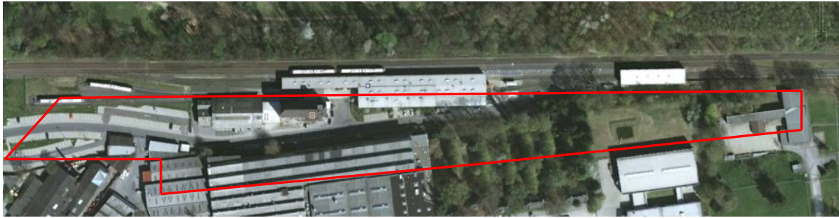
Figure 5-19: Example: Depot and Workshop area for 14 DMU's, REGIOBAHN Dusseldorf, Germany (approx. 550 m * 25 m)
