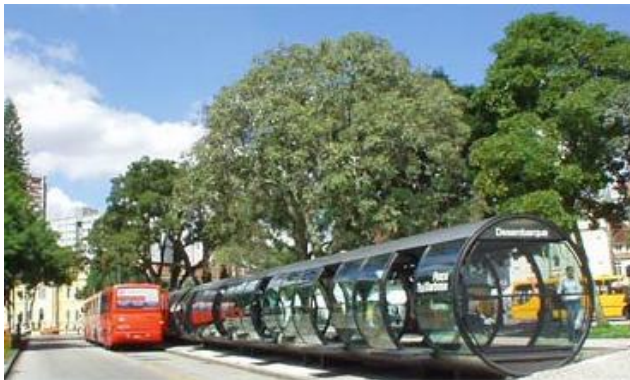
Figure 5-26: Example 3 Station BRT Curitiba Station,
