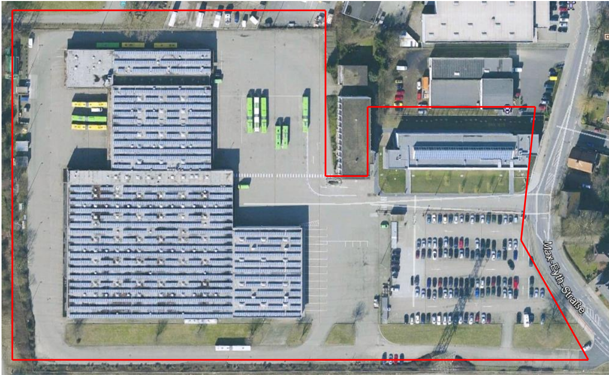
Figure 5-31: Example: Bus depot and workshops for 120 buses, Oberhausen Germany (approx. 250 m * 170 m)
