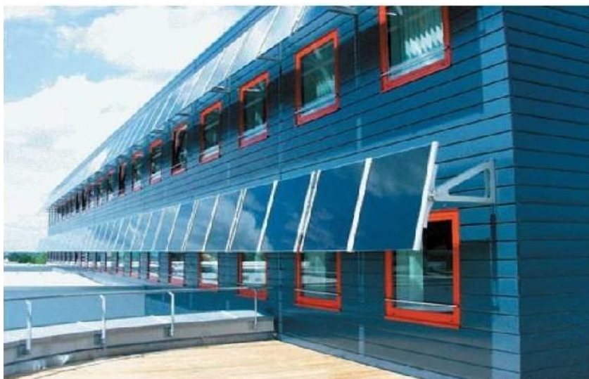
Figure 60: Modules photovoltaïques brise-soleil
