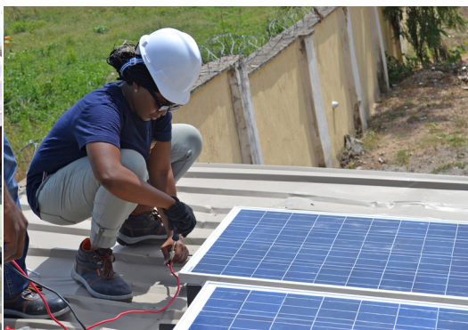
Photo left: Training on new developed Standards for Solar PV Components
