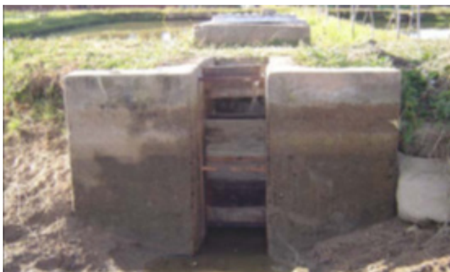
Fig 3.28 a monk used as an outlet and overflow
