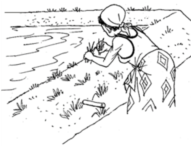
Fig 3.34 and Fig 3.35 pond dykes planted with grass
