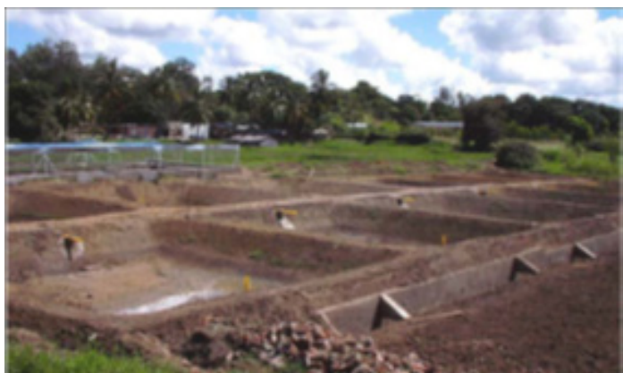
Fig 3.1 a Paddy ponds showing inlets
