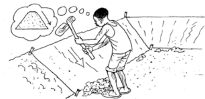
Fig 3.21 shaping inside pond slopes Fig 3.22 levelling and slopping the pond dykes
