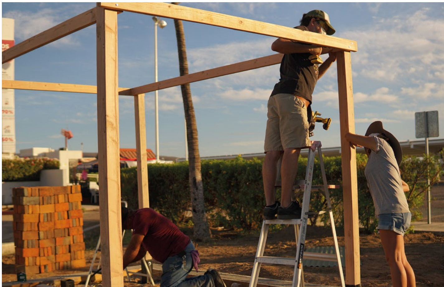
Construction of urban facilities ©Alianza Oasis Urbanos.
