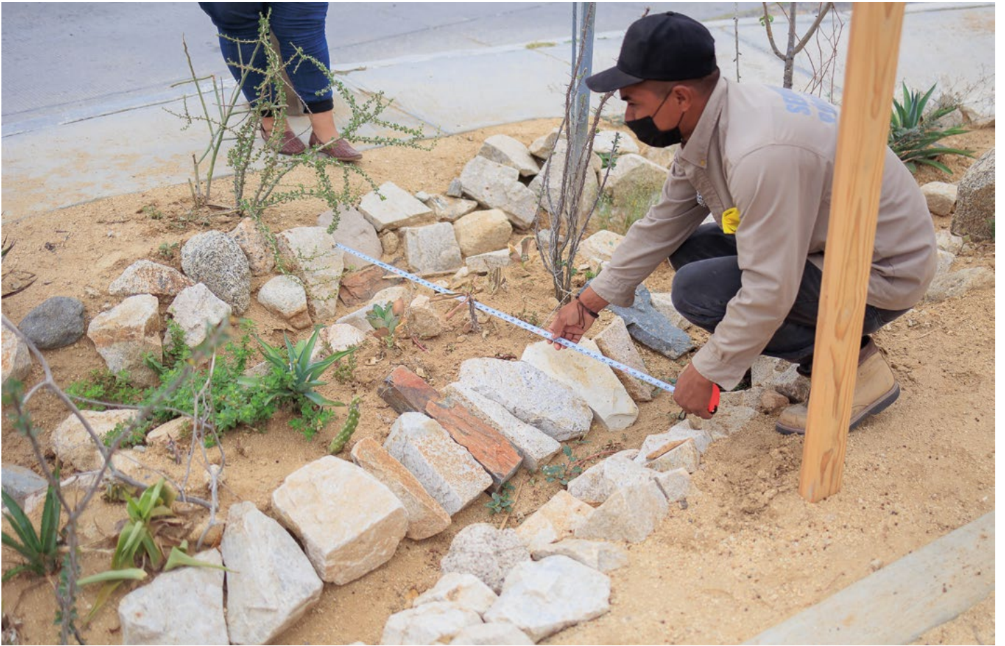
Measuring the dimensions of a micro-basin ©GIZ México, Josafat de la Toba.
