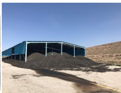
Left: Sludge Drying Beds in Wadi Mousa Wastewater Treatment Plant
