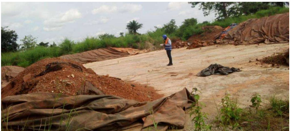
Image 10: Storage space for contaminated waste rock
