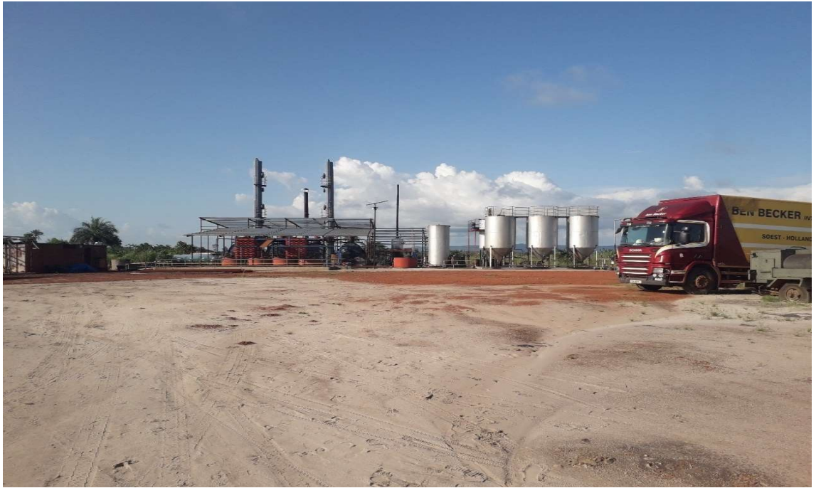
Image 22: Oil recovery unit at Tanènè
