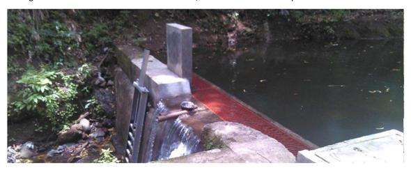
Figure 12. Improved water intake at Mont Reuil water intake ("Tyrolean weir" type grille with slatted horizontal water intake pipe inside the weir)
