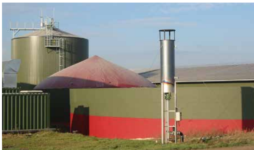
Gas flares safely release excess pressure.
