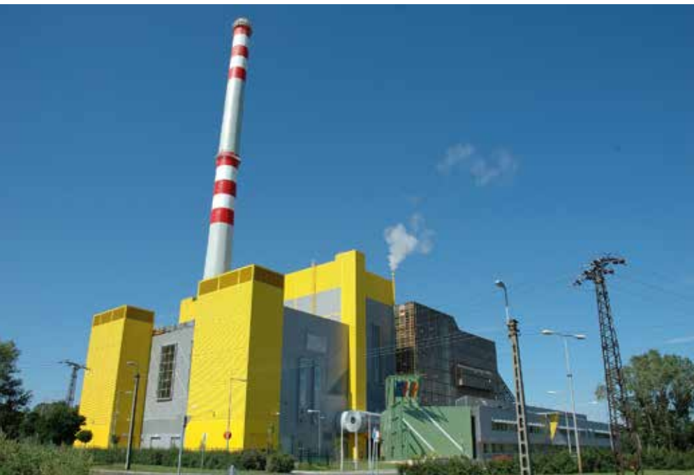
A municipal solid waste incineration plant in Europe.
