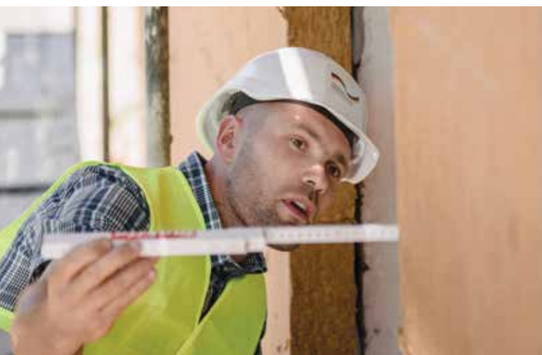
Ukrainian workers are renovating public buildings
