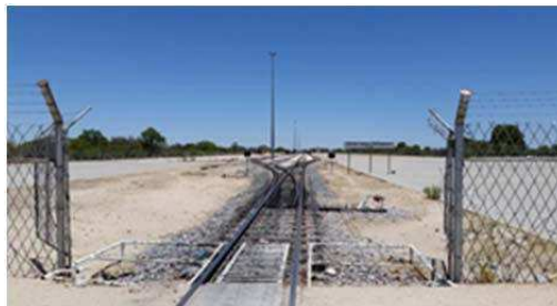
Figure 11: Railway freight station at the border in Oshikango
