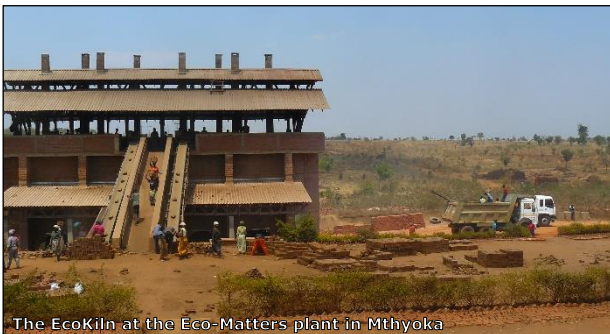
The EcoKiln at the Eco-Matters plant in Mthyoka
