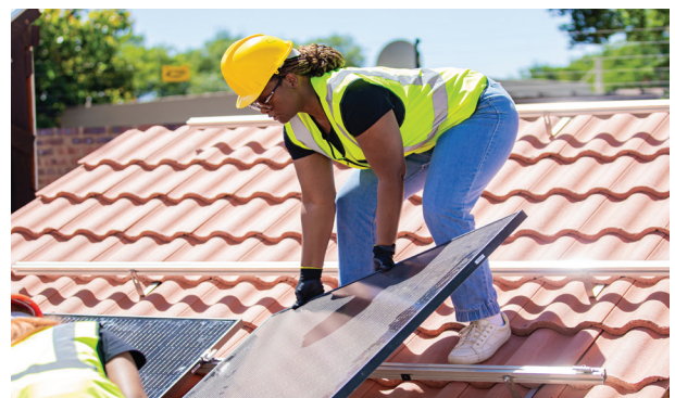
Learners are installing solar panels at a Training Centre in Benoni, Johannesburg
