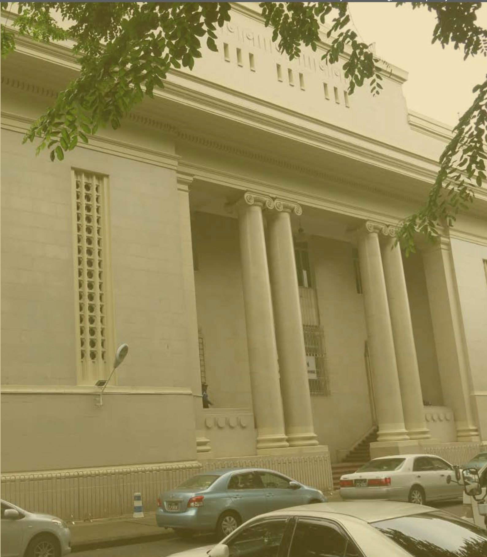
Former Central Bank of Myanmar building, Now occupied by YSX
