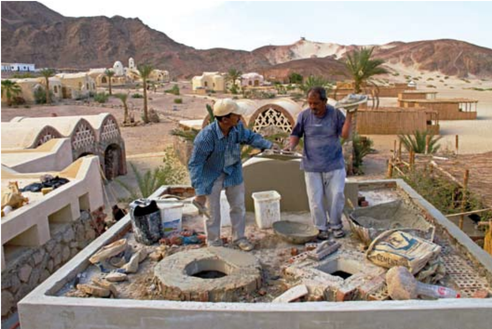
© M. Seyppel. Two workers are building an energy-efficient and climate-friendly house.
