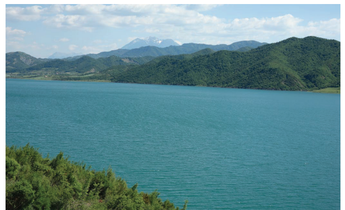
L. to r.: Peqin: private cisterns on the roof - Water supply dam in Banja near Cerrik
