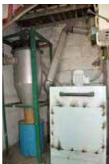
FIGURE 6: E-WaRDD cyclone and dust collector © E-WaRDD 2010
