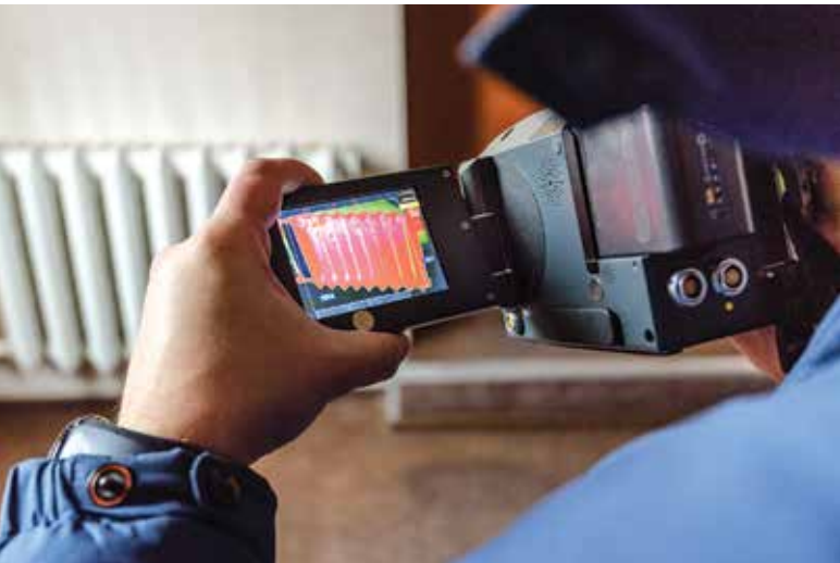
Checking a radiator with a thermograph
