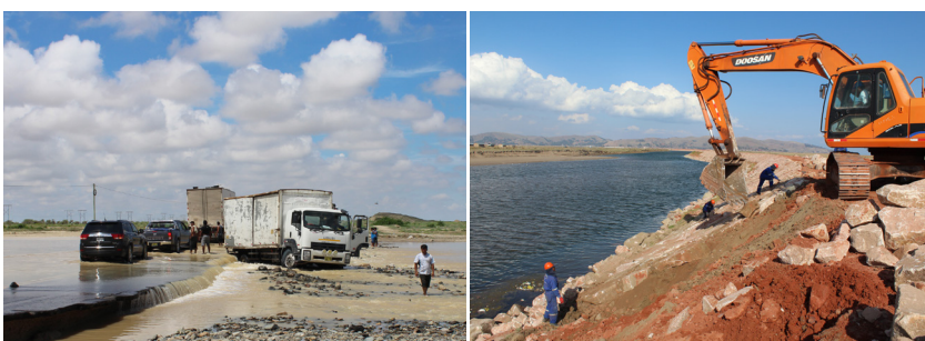
Left: Extreme weather events can damage public infrastructure and lead to the blocking of important traffic axes.
