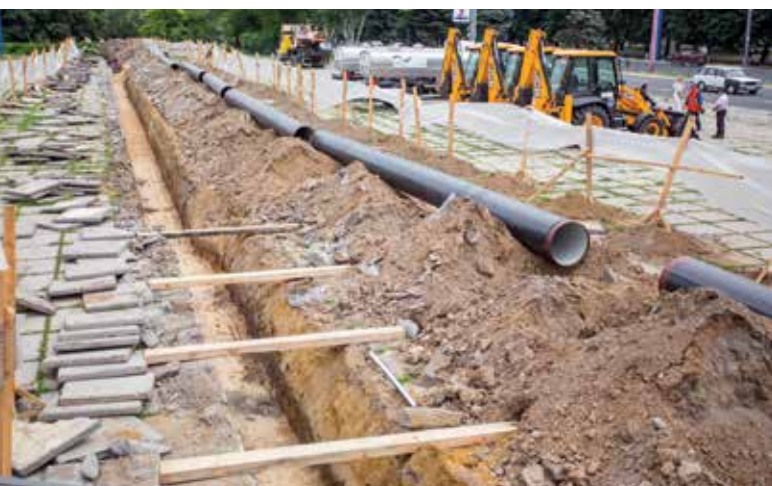
Repair works on water pipes in Mariupol
