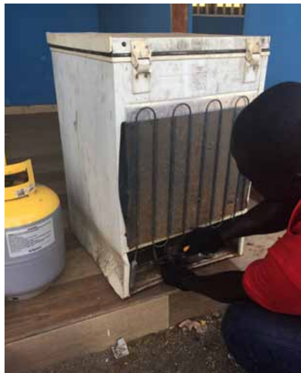
Good Practice: Extraction of cooling gases before fridge dismantling for recycling (Ghana) ©WRF
