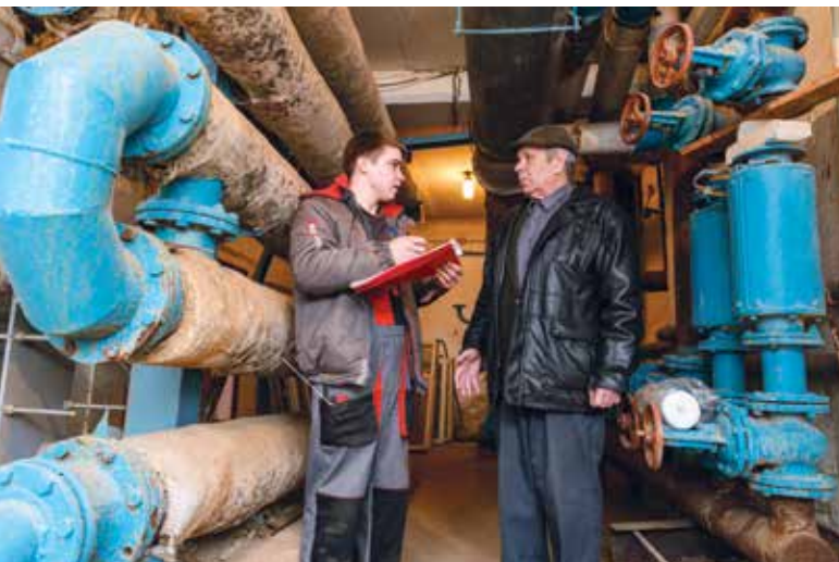
Inspection of heating systems
