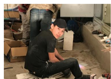
Construction workers in the Ger district of Ulaanbaatar @giz/Töpfer
