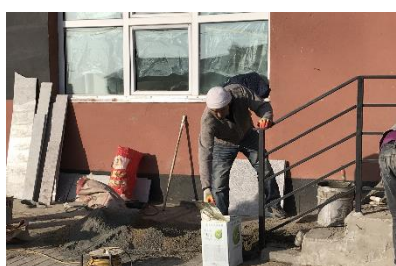
Construction workers in the Ger district of Ulaanbaatar @giz/Töpfer
