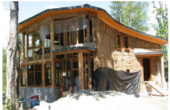
Building a straw-bale house, Designed by Carina Rose. Author Colin Rose https://commons.wikimedia.org/wiki/File:Straw_Bale_House06.jpg
