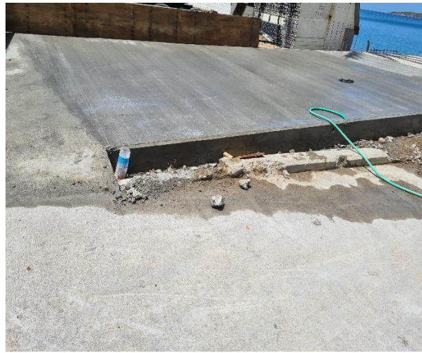
Finished ramp extension for ease of access
