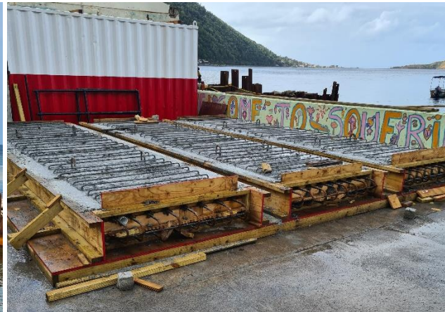
Curing of slabs prior to installation on jetty platform
