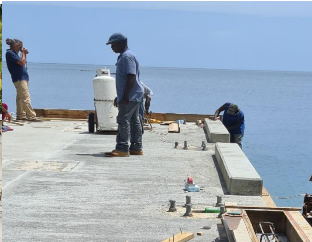
Completed curbs for jetty
