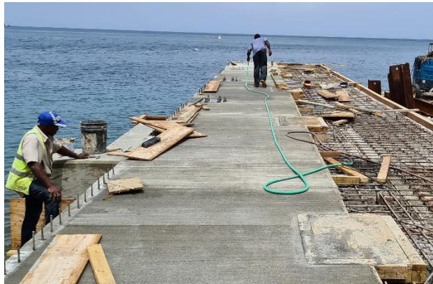
Wetting of pored surface to prevent cracks
