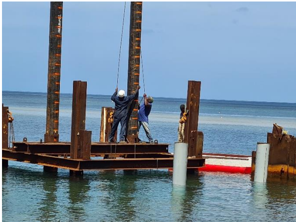
Installation of additional coated piles
