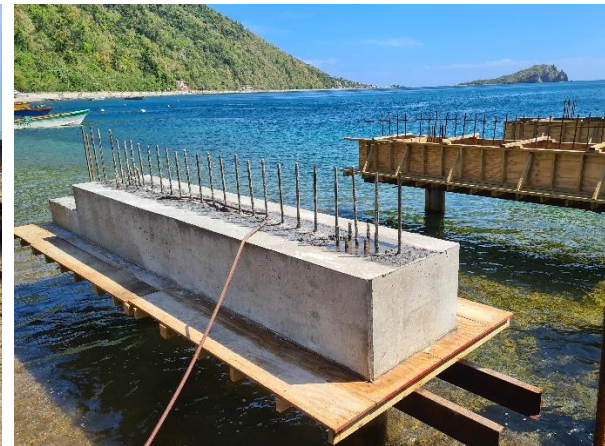
Example of completed capping
