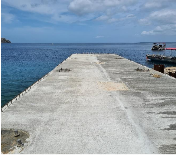
Completed jetty surface without ramps
