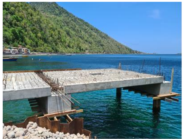
Completed capping with slabs installed
