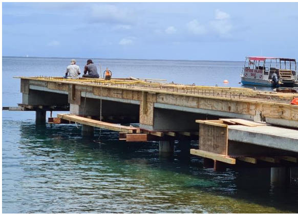
Formwork of slabs and landing edge for concrete in progress
