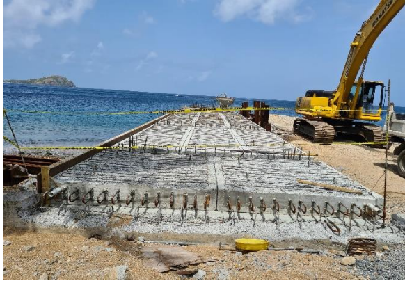
Slabs in place on all capping awaiting remaining steelwork before surfacing
