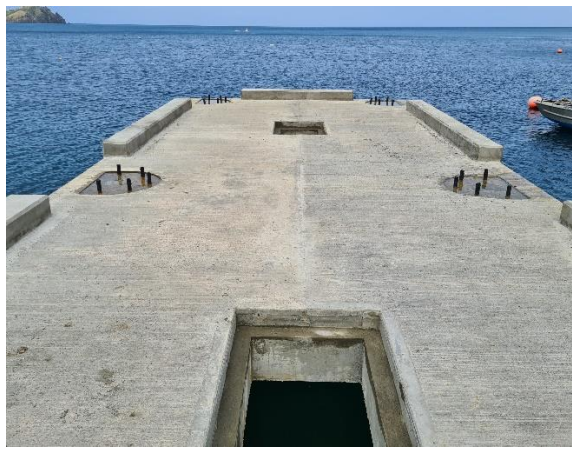
Blow hole to dissipate wave energy and uplift
