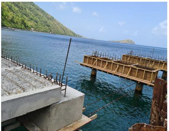
Precast slabs placed on finished cappings
