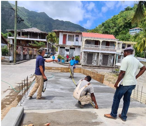
Inspection of the facility
