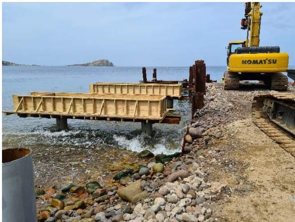
Capping form works in progress
