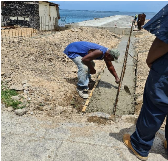
Construction of jetty ramps system underway
