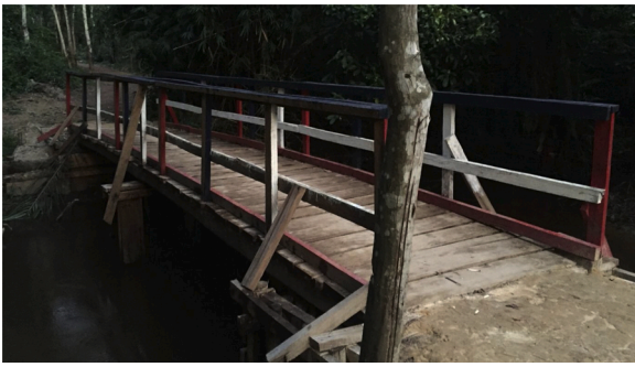
Fig. 5. Newly-Constructed 'Engineered Timber Bridge' in the Gogein Study Area.
