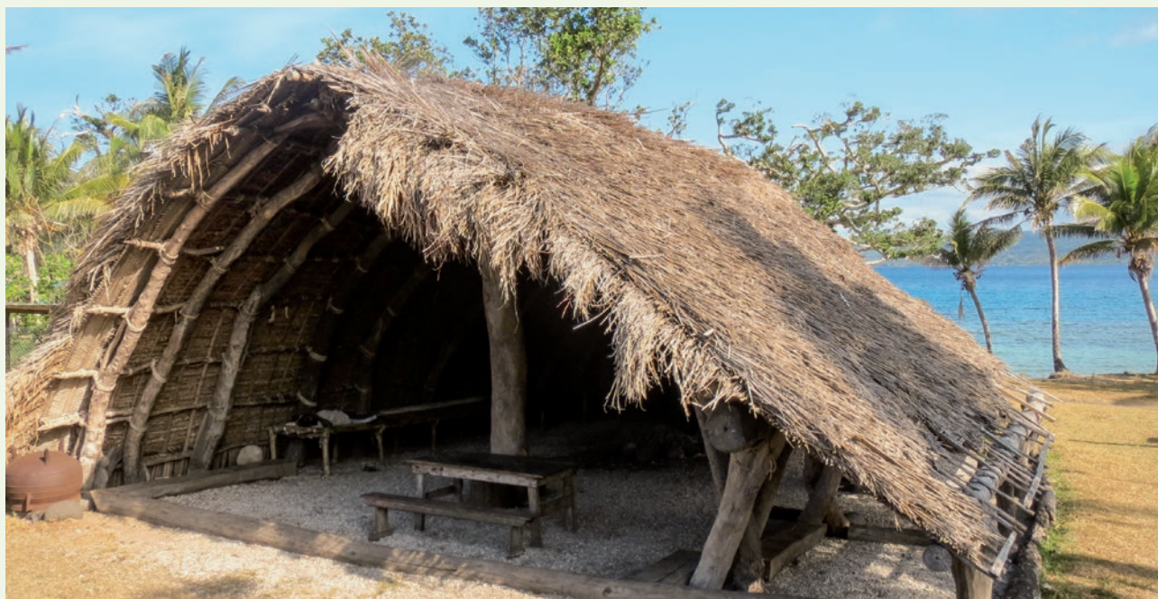
Figure 7: The nakamal in Taloa, made from local materials, appears solid and safe. It provided shelter mainly to young men from the community and suffered only minor damage during the cyclone.
