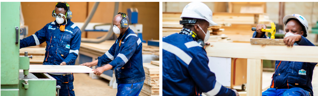
L to R: Carpenters polishing wood before building a door; Carpenters putting together a wooden door
