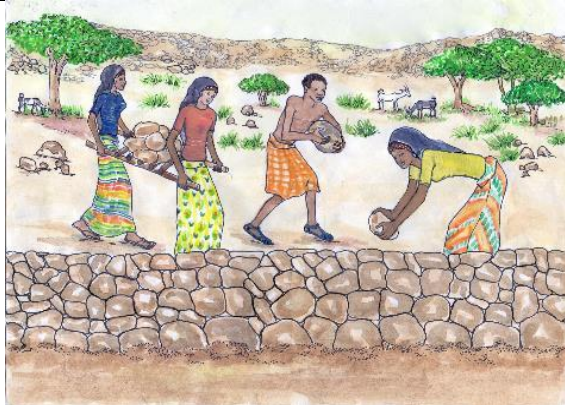
Fig. 4: Drystone Structure, almost finalized. Community team members bring big flat stones to cover the small stones
