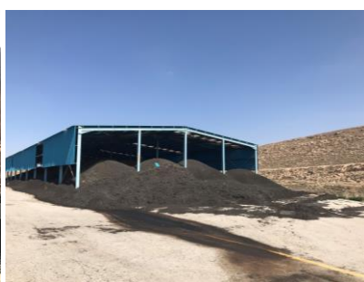
Left: Sludge Drying Beds in a wastewater treatment plant
