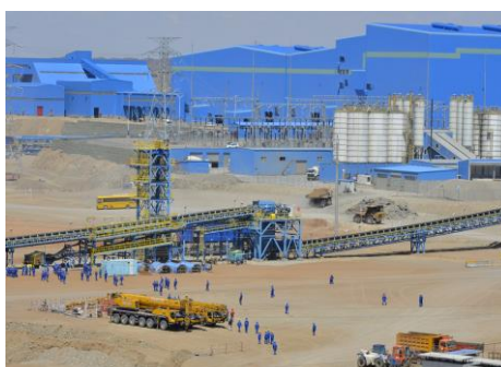
Photo (L) to (R): Engineers at a construction site
