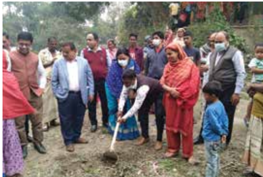
Earth filling work inaugurated by the Mayor of Sirajganj Municipality
