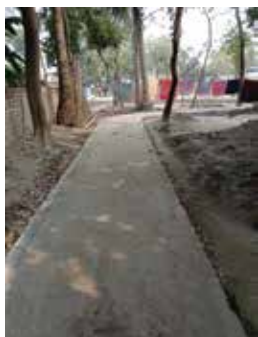
Road after construction
