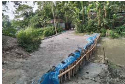
After earth filling, the road is visible
