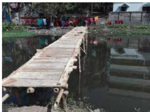
Wooden bridge is in under construction
