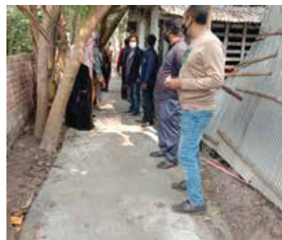
Members of the core team visiting the constructed road.
