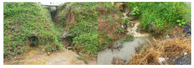
Figure 13: Examples of required drainage improvements (Highway 317 (L), Highway 3193 (R))
