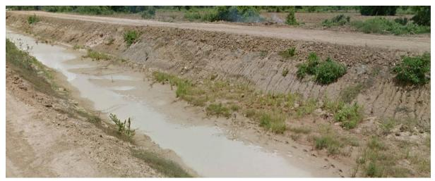
Figure 29: Signs of erosion of canal banks and sedimentation
