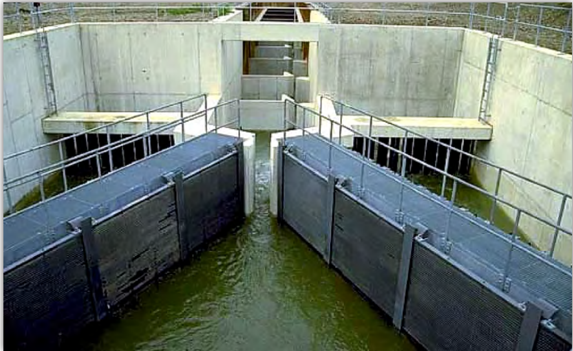
Figure 50: Fish screen at Iffezheim Dam, Rhine River looking downstream
