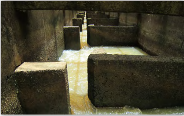
Figure 26: Inside the vertical-slot fish pass at Stung Chinit Weir looking upstream
