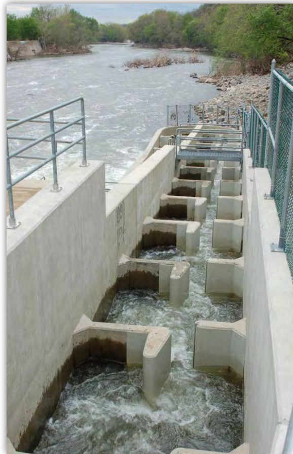
Figure 27: A typical vertical-slot fish pass looking downstream
