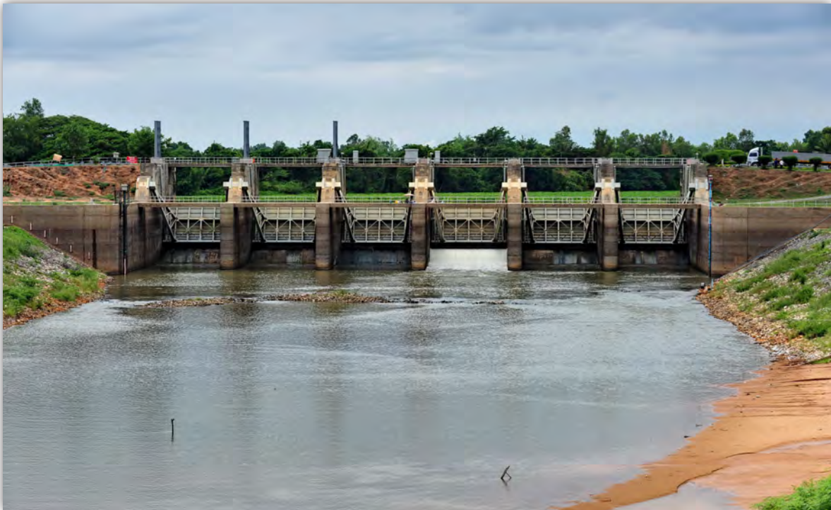
Figure 13: Khuoi Cheua Weir on the Chi River in northeast Thailand
