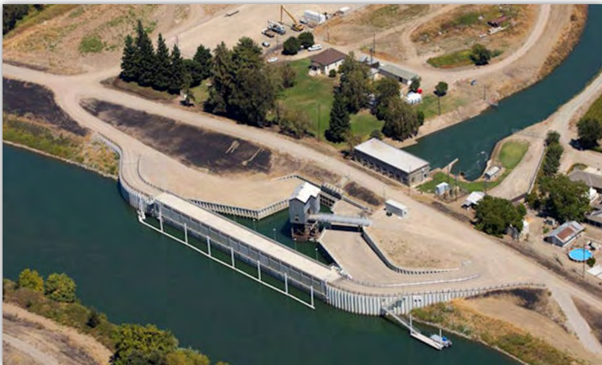
Figure 49: A wire-mesh screen prevents fish passing into a diversion channel
