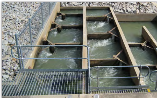
Figure 28: Vertical-slot fish pass at Lock 10 on the Murray River, Australia
