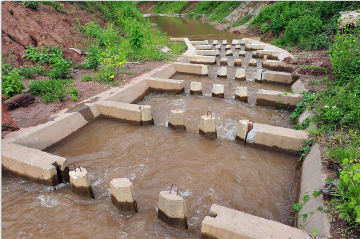
Figure 29: A recently constructed cone fishway in Lao PDR
