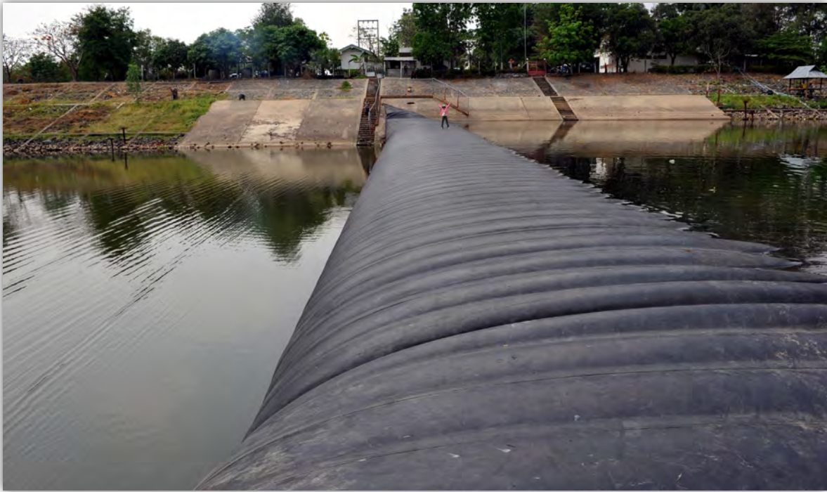
Figure 8: One of several rubber weirs across the Mun River, Thailand
