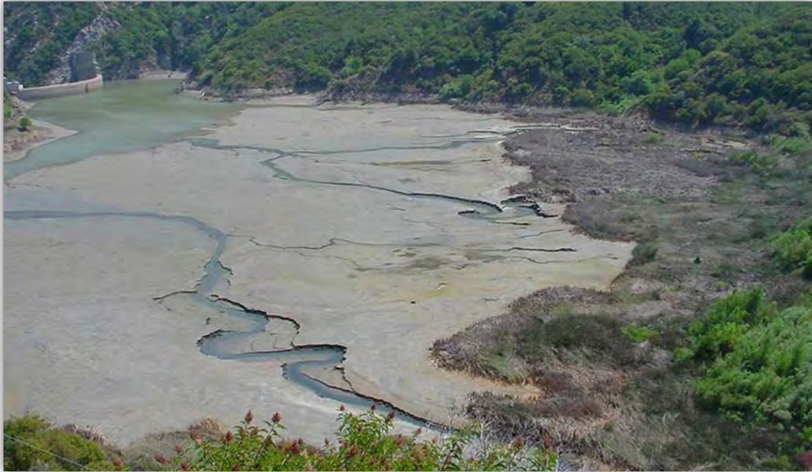
Figure 61: Matilija Reservoir in California, showing extreme sedimentation
