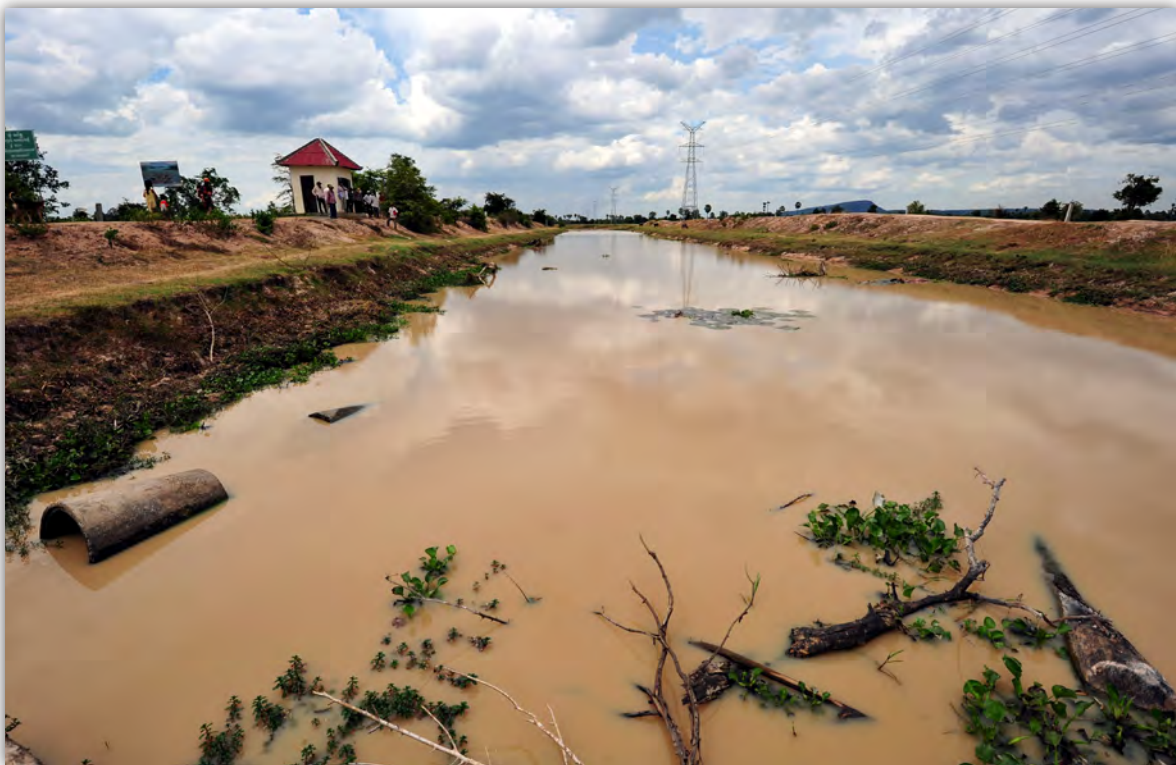
Figure 11: Boeng Chertrao, a typical small irrigation reservoir in Cambodia The bed of the stream has been excavated, with the clay spoil used to make a dam wall. Photo: Kent Hortle
