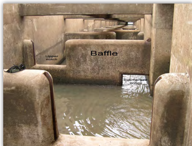
Figure 23: Inside a pool-and-weir fish pass at a dam on the Mae Nam Kham River Thailand
