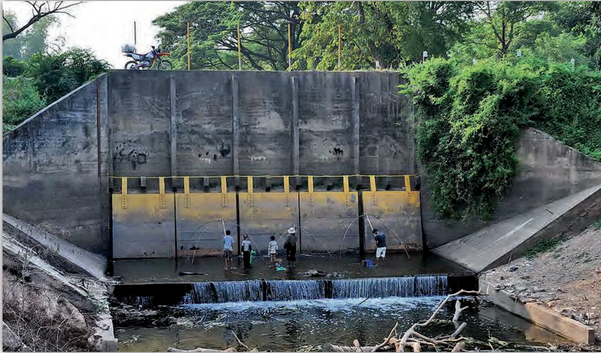
Figure 92: A prime site for improving fish passage – a regulator on a small tributary
