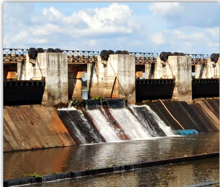
Figure 39: Tumnub Makak Dam, Kampong Thom, Cambodia
