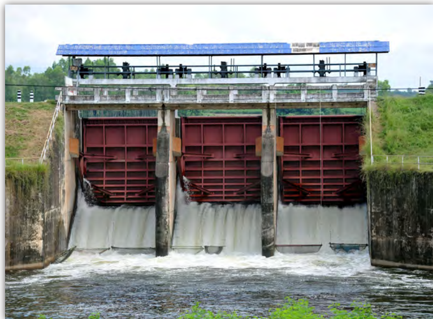
Figure 37: Typical top-down radial water gates, Huai Luang Dam, Thailand
