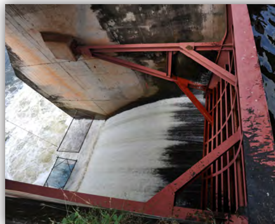
Figure 37: Typical top-down radial water gates, Huai Luang Dam, Thailand
