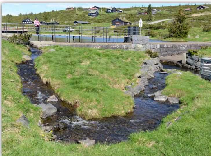
Figure 35: A nature-like bypass fish pass at a small weir
