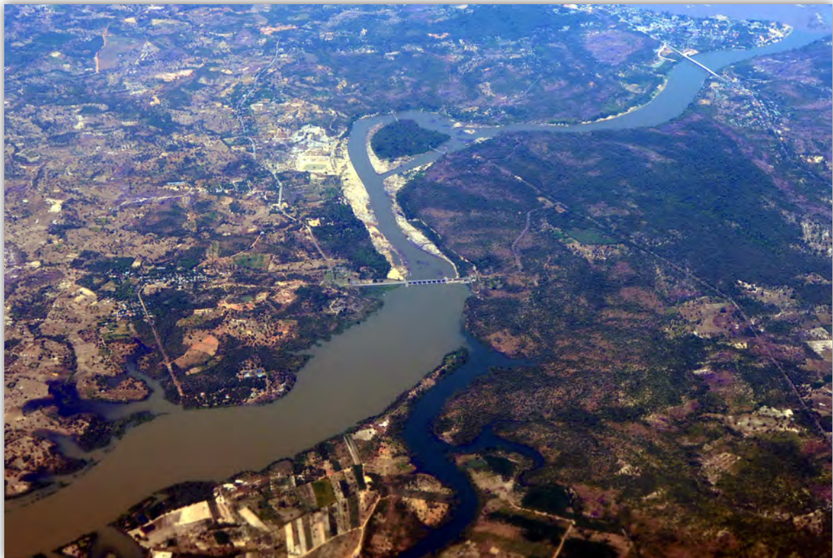
Figure 7: Pak Mun Dam in Thailand, a ‘run-of-river’ hydroelectric dam
