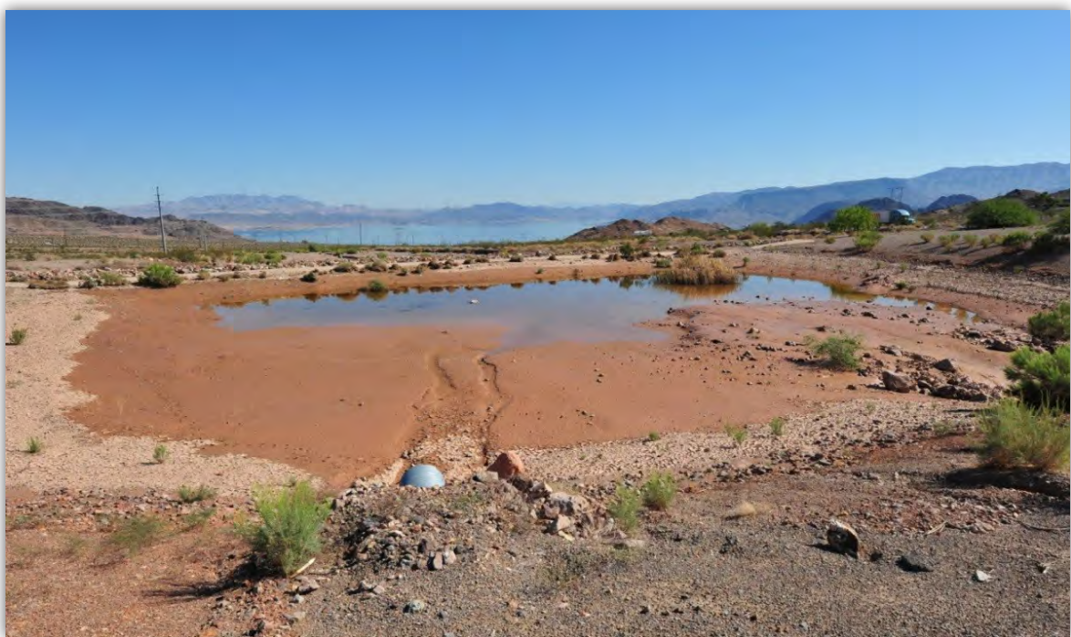
Figure 64: A trap reduces sediment input to Lake Mead, the reservoir of Hoover Dam, USA Control of sediment reduces reservoir sedimentation, and also reduces turbidity, allowing light to penetrate, which increases aquatic productivity.
