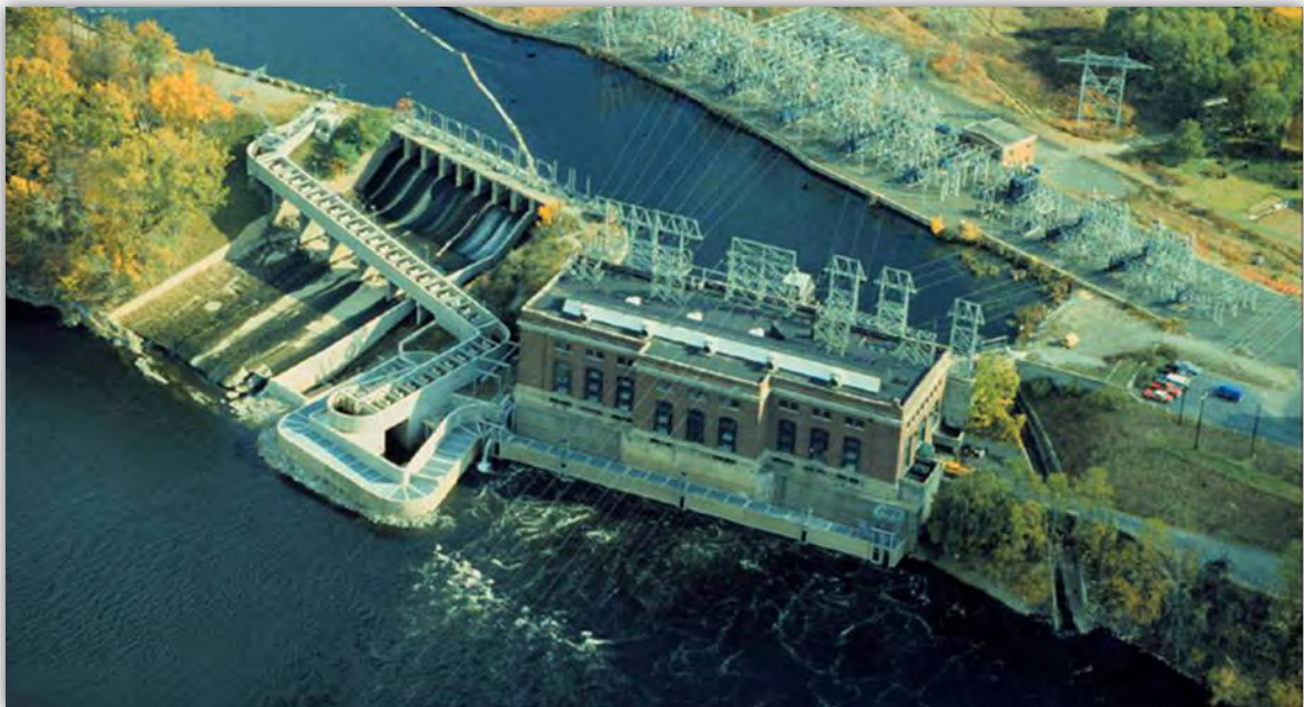
Figure 36: A pool fish pass at a small hydroelectric weir
