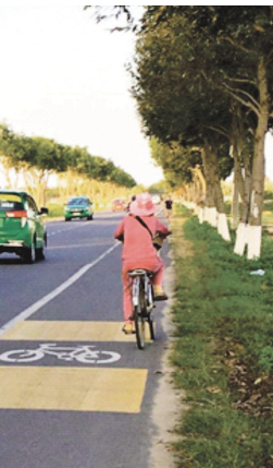
Figure A.1. Dedicated bicycle lanes separated by markings on the Hai Ba Trung route, Hoi An (Source: GIZ TUMI Project Hoi An)
