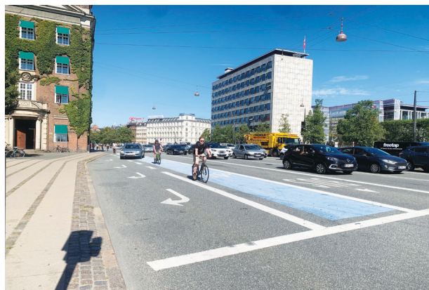
d) Unprotected bicycle lanes at the intersection. Bicyclists feel much less confident in comparison with the case in photo c
