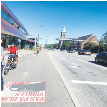
c) Bicycle lanes are protected when approaching the intersection, bicyclists feel confident
