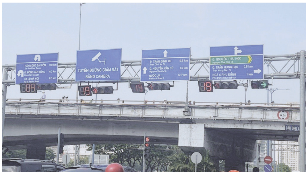
Figure 6.1. Signal heads for each traffic lane
