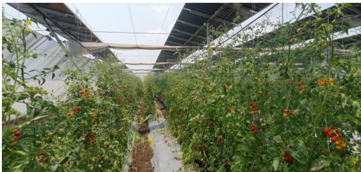
1.4 MW Agrivoltaic plant in Parbhani, India © IGEF-SO, GIZ India
