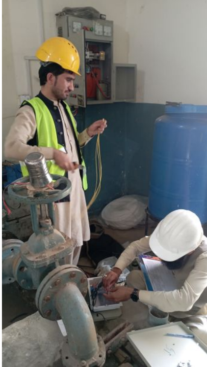
Energy Management System Installation © GIZ Pakistan
