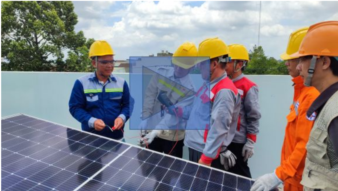
Parameter measurements under normal operating conditions and changing conditions © GIZ/ESP
