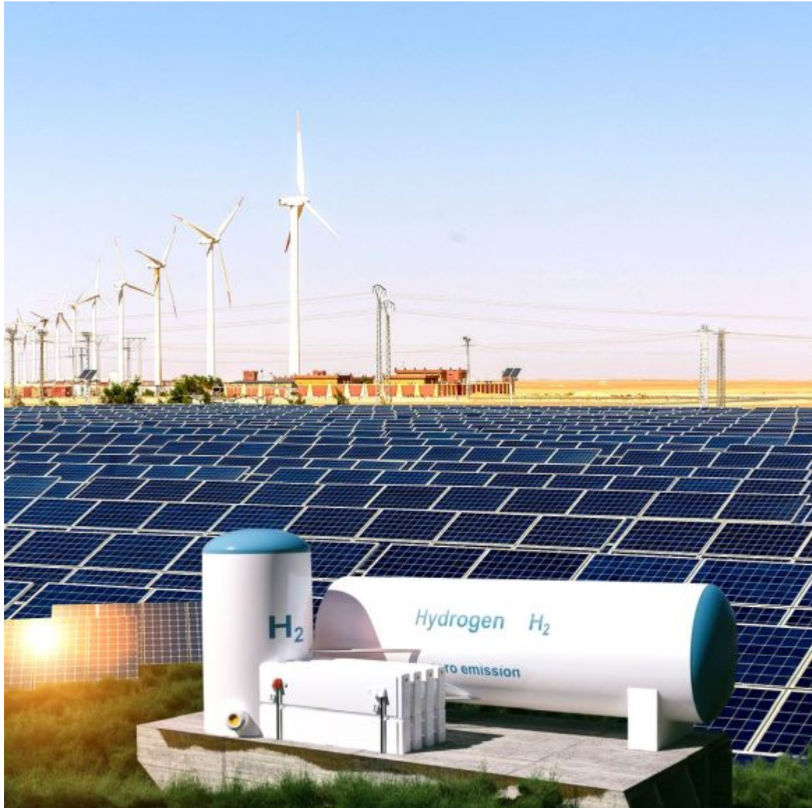
PV and wind turbines Plant in Adrar/Algeria © Taqat'Hy Project
