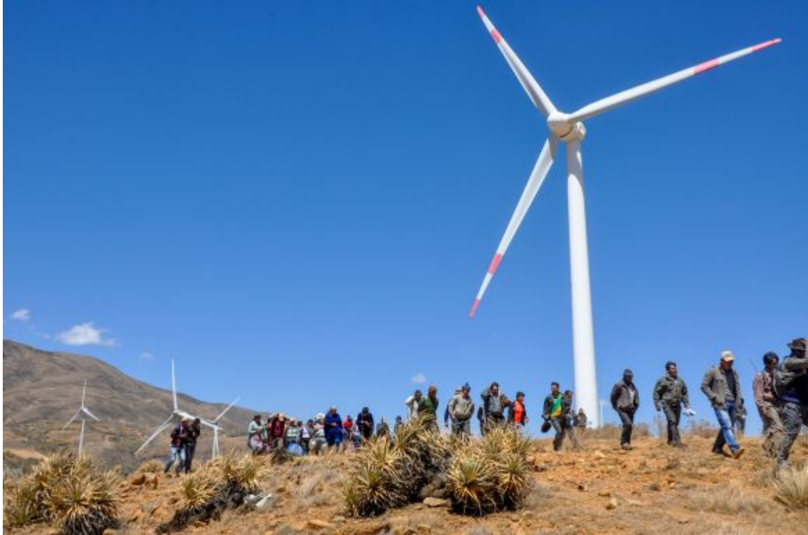
Qollpana wind farm. Cochabamba, Bolivia © PEERR/GIZ
