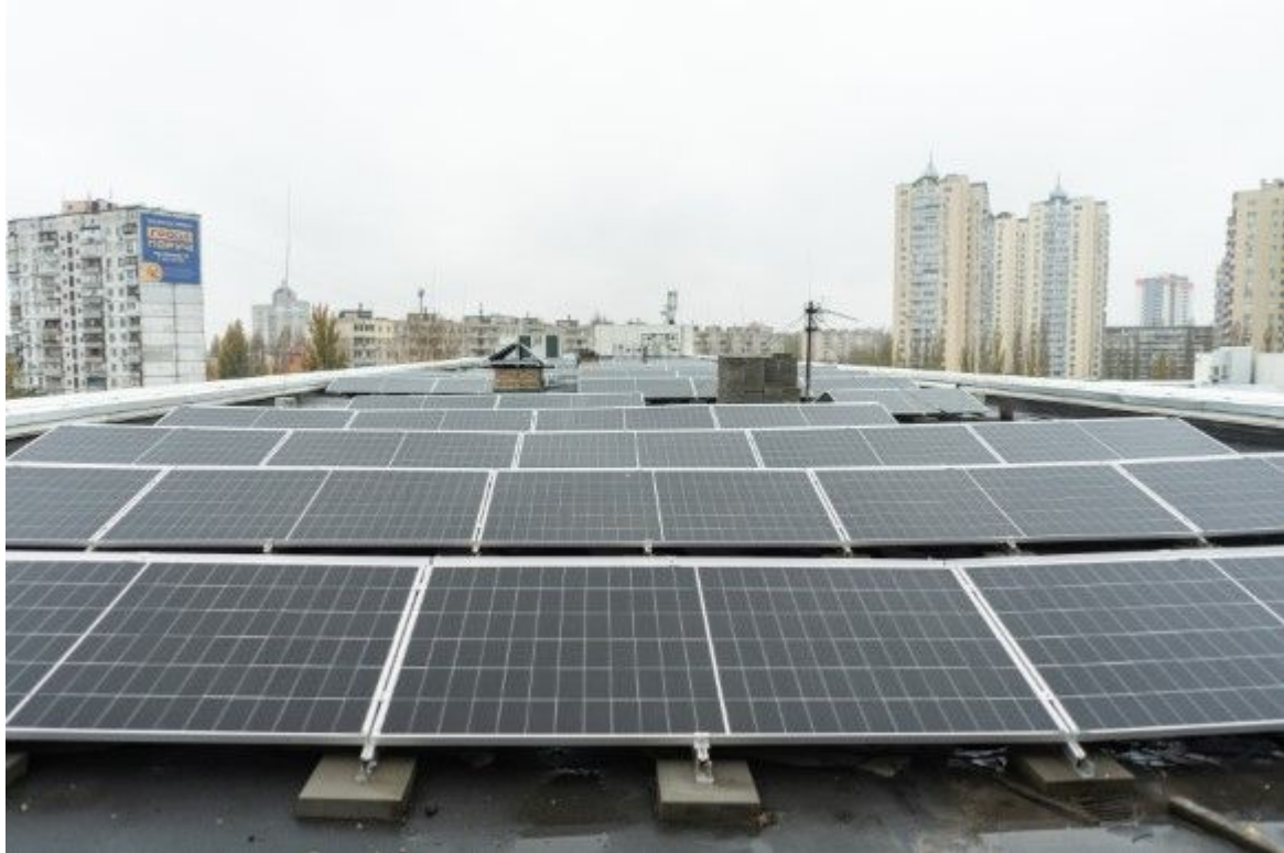
Solar power station on the roof of the hospital © the gate agency
