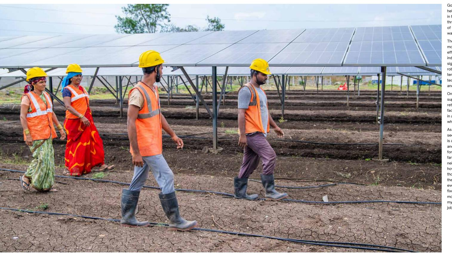
Govind was right. While transpiration by the plants helps in keeping the solar panels cool, aiding in their maintenance, the plants are irrigated through solar water pumps. Planted in the shade of the solar panels, these plants also require less water since not too much is lost to evaporation.
