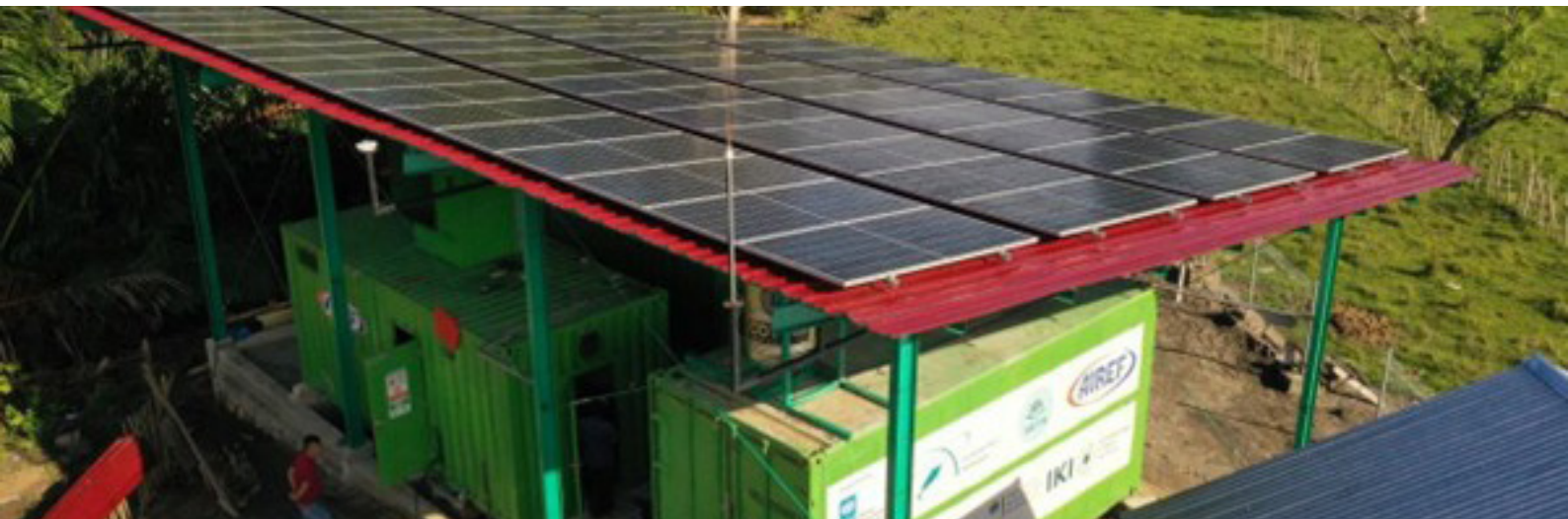
FIGURE 4 | Solar Ice Maker in Kawa, powered by a 27 kWp solar PV installation.
